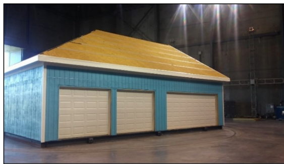
(a) Test house with twin-single and double doors on the "west side".
